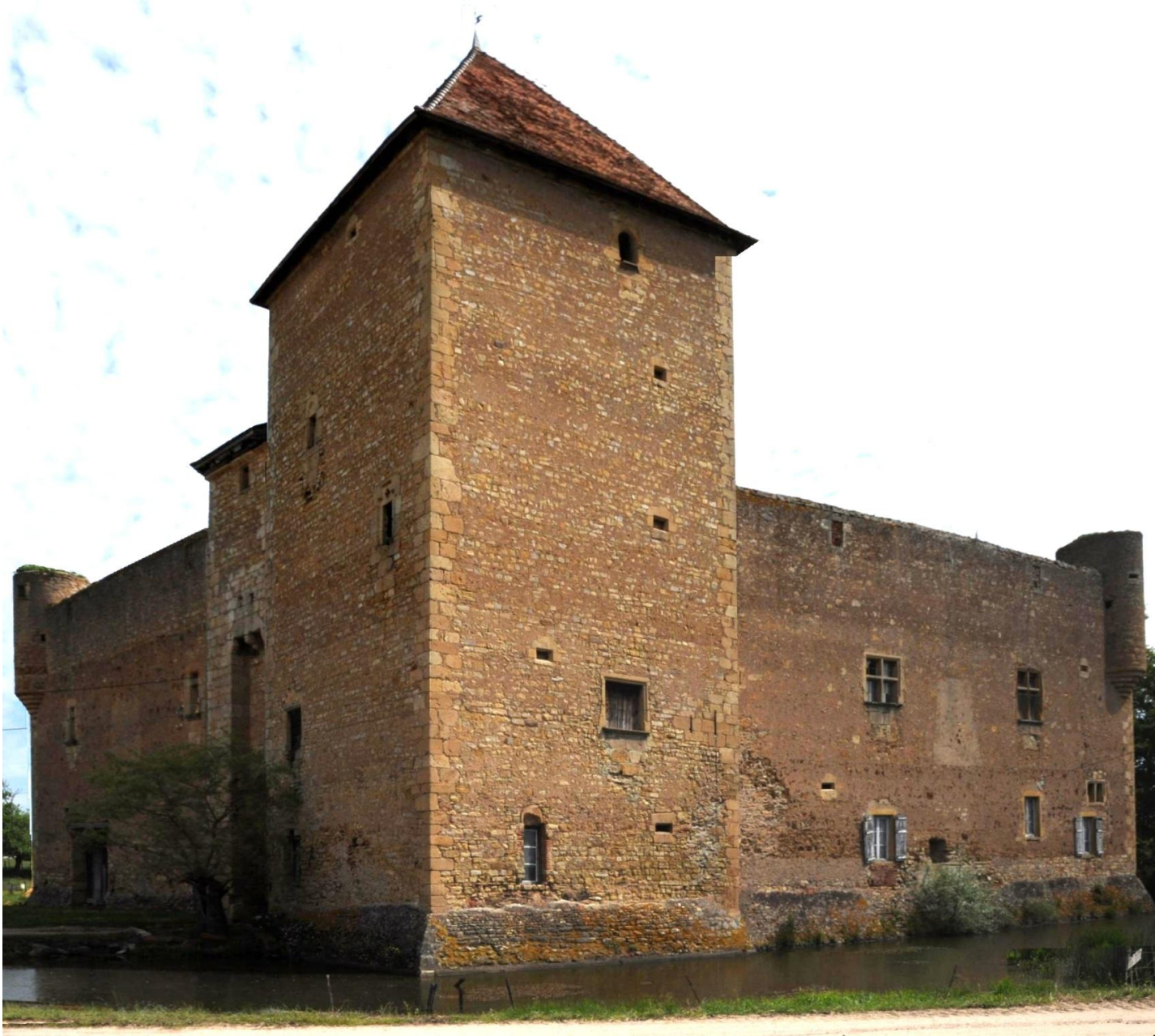
© photo M. Jalabert 2013
